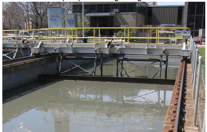
Primary Skimmer at East Providence Treatment Facility
