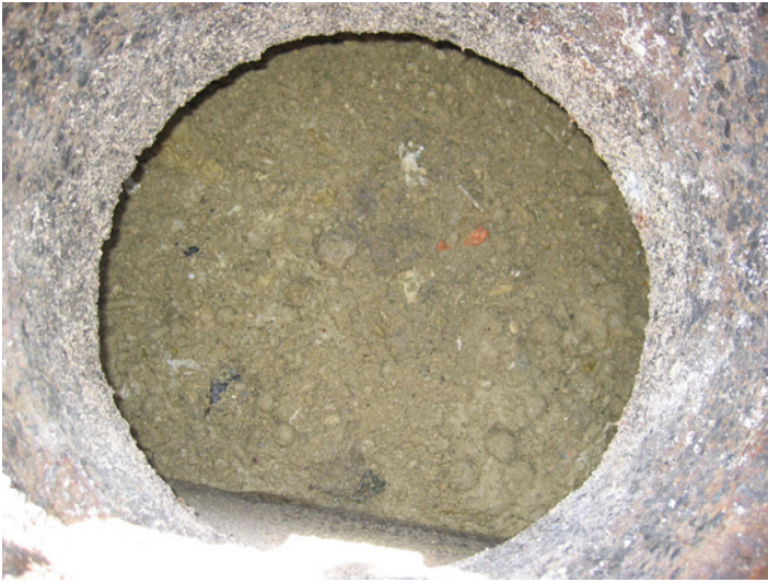
Grease pit at East Providence treatment facility
